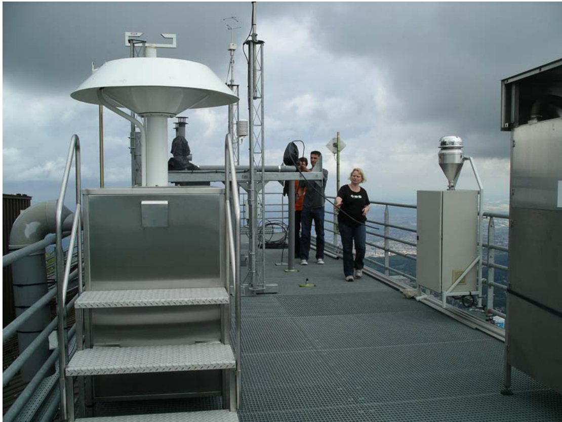
Work in progress at Put the Dome Station...
