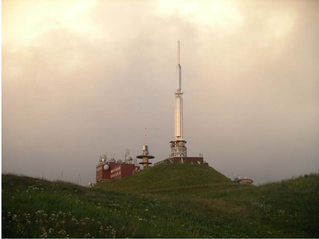
Puy de Dome Station
