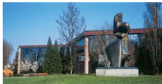
External view of the Palais des Congres in Strasbourg.
